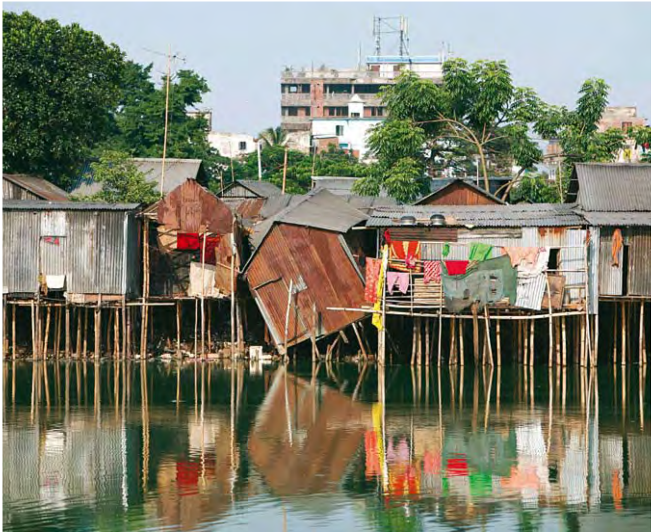
▲ Raised slum dwellings built near the banks of the River Buriganga, Dhaka, Bangladesh. Cities in river deltas are particularly vulnerable to flooding. ©Manoocher Deghati/IRIN
